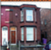
Alderson Road L15
