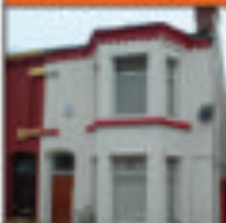
Alderson Road L15
