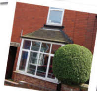
Derham Road 6 Houses
