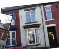
Harefield Road, S11 3 Bedroom Terraced House
